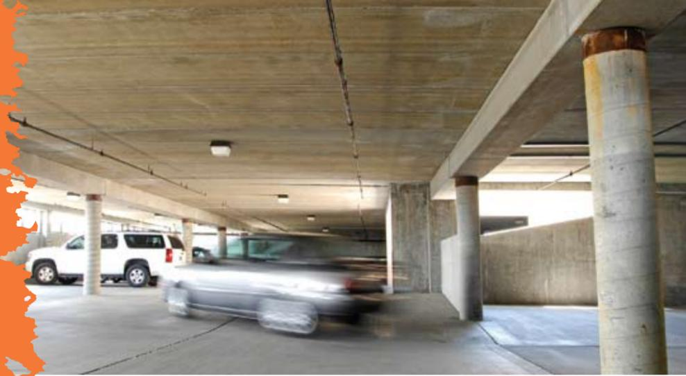
**Precast Platform Buildings** are best described as a precast concrete solution that works in conjunction with wooden constructions up to four stories in height.
